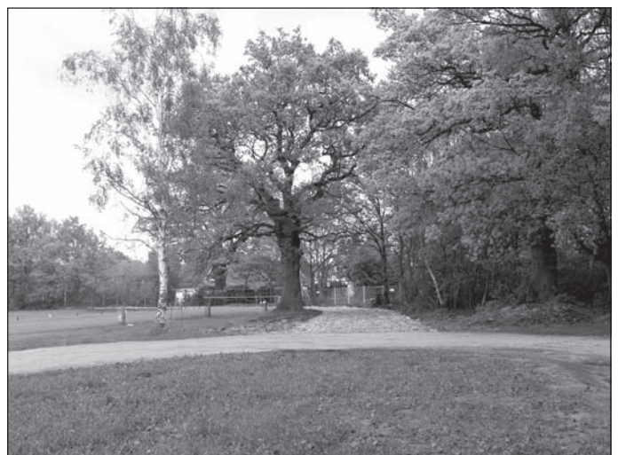
Hobson's Way - the new road in its final stages of construction.
