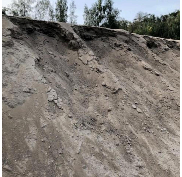
Example of tunnelling in a sand stop butt prior to de-leading.
