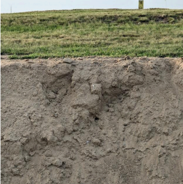
Example of tunnelling in sand stop butt prior to de-leading.
