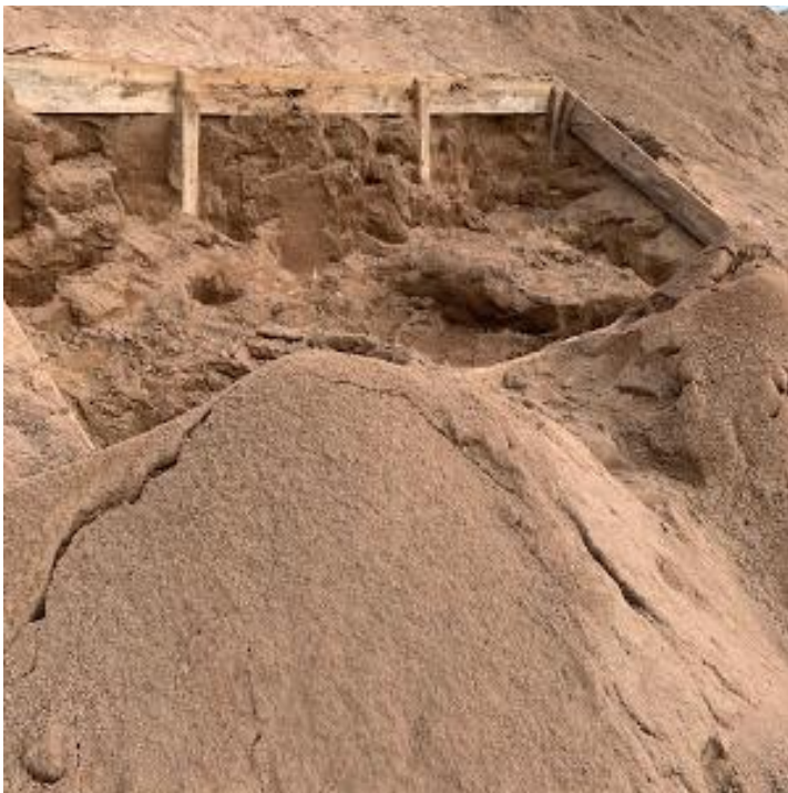
The Butt stop sand is sieved, checked and all ricochet hazards removed
