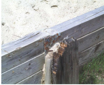
Figure 5 - Here the timber protection has been shot away exposing firers to backslash from a metal plate
