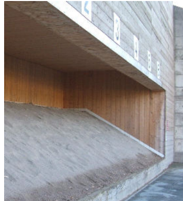
Figure 3 - Marking the 34 deg slope where it is possible to do so is good practice
