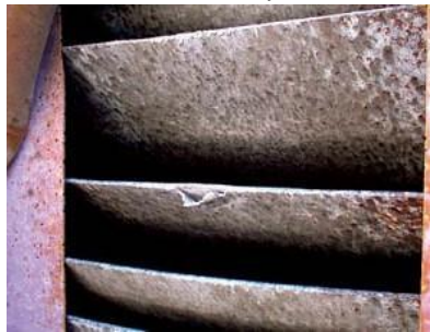
Figure 14 - Venetian Blind Bullet Trap system
