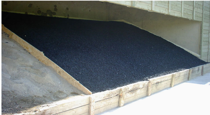
Figure 10 - Granulate Bullet Catcher on a Barrack Range
