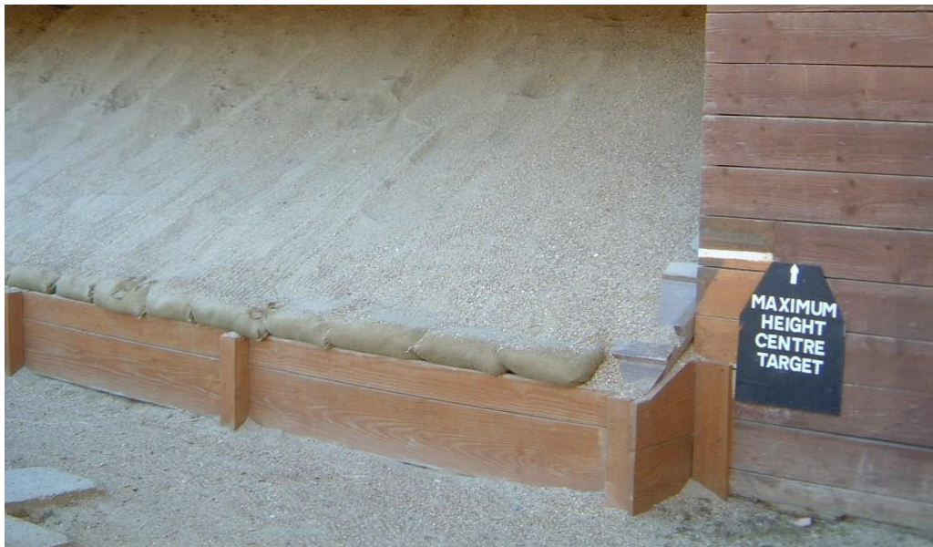
Figure 6 – Target Centre Height (TCH) Marking
