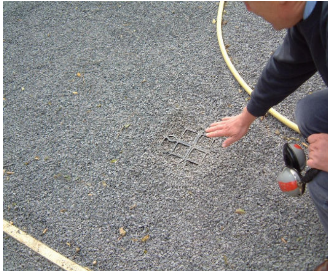
Figure 7 - Plastic grid used to form gravel path
