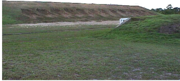
Figure 2 - A poorly maintained gallery stop butt with too much scooping
