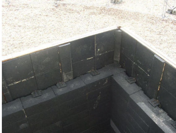
Figure 13 - Dense Rubber Block and Tile Bullet Trap system
