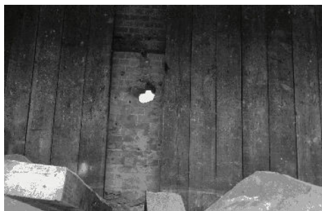
Figure 4 - Here timbers have been removed to check the back wall
