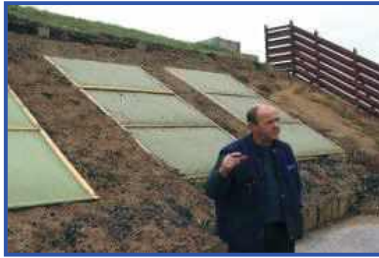
Figure 9 - Example of rubber granulate shooting in boxes on the stop butt. (Hessian cover keeps the granulate in)
